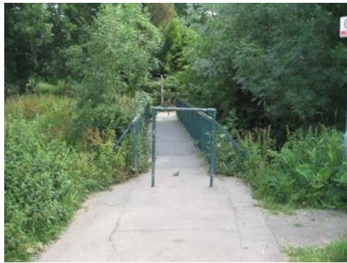
Site of new Hogsmill cycle bridge to be installed in 09/10 as part of current Greenways programme
